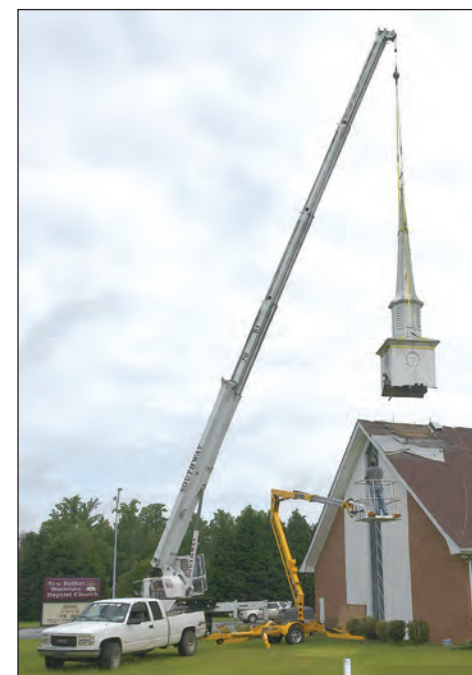
A crane operator removes a steeple from New Bethel Missionary Baptist Church in 2017.
