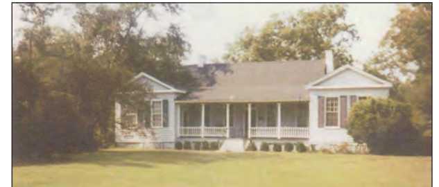
The McQueen house still exists on the corner of Hampton Avenue and McQueen Street.
