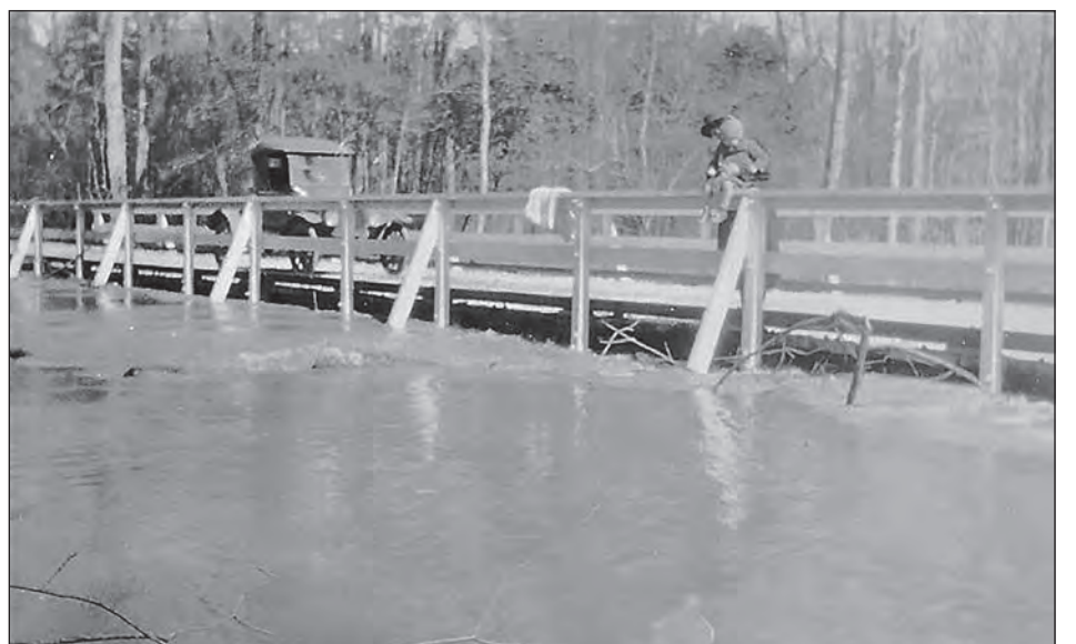
The bridge over the Wateree River is seen under construction during the 1920s. A “spring freshet” had the water level up to the bridge. Bridge engineer Ambrose Gonzales is seen standing on the bridge.
