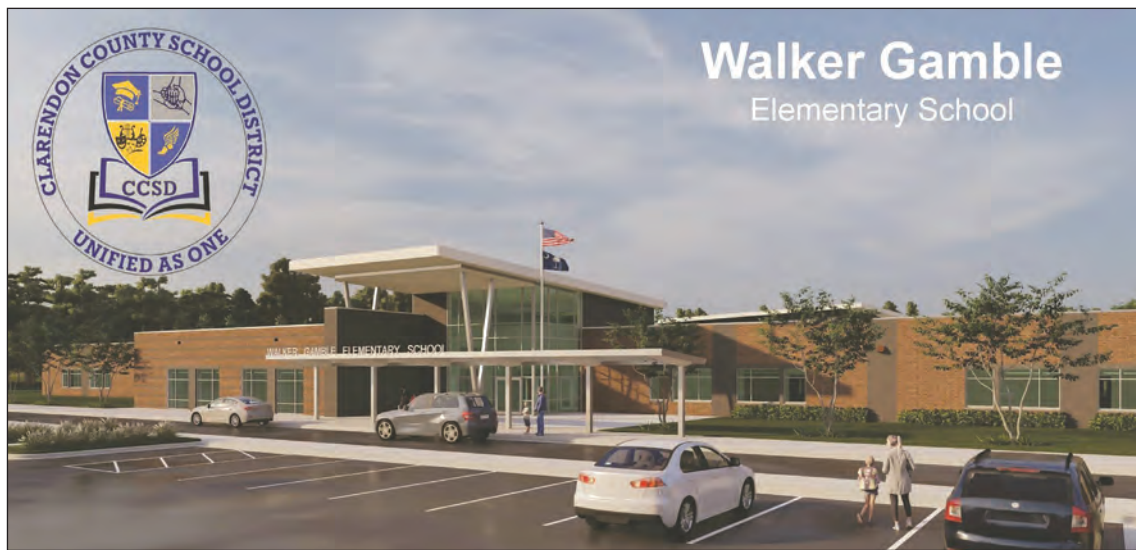
The new Walker Gamble Elementary School is expected to be completed in 2025.
