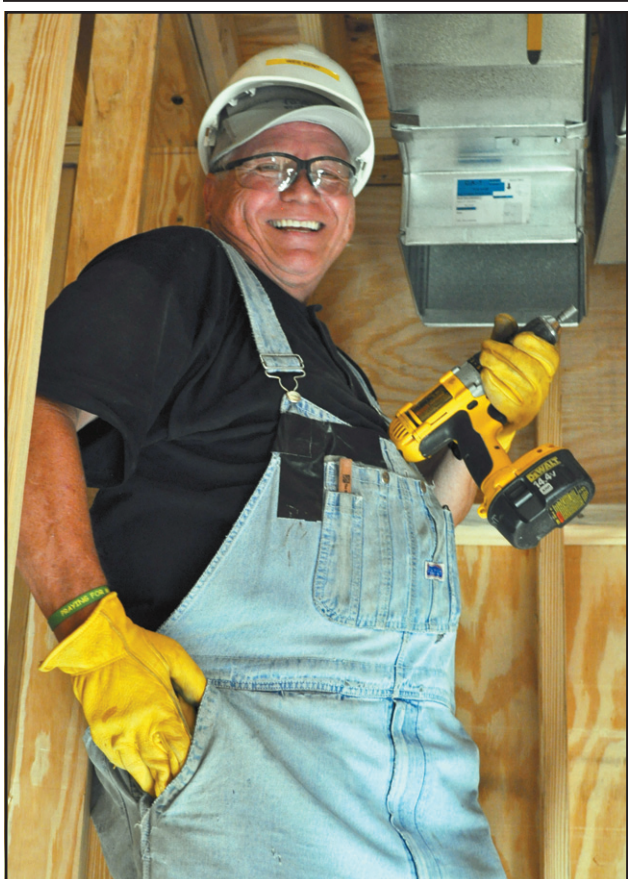
The late Wes Kent installing ductwork on a building project.
