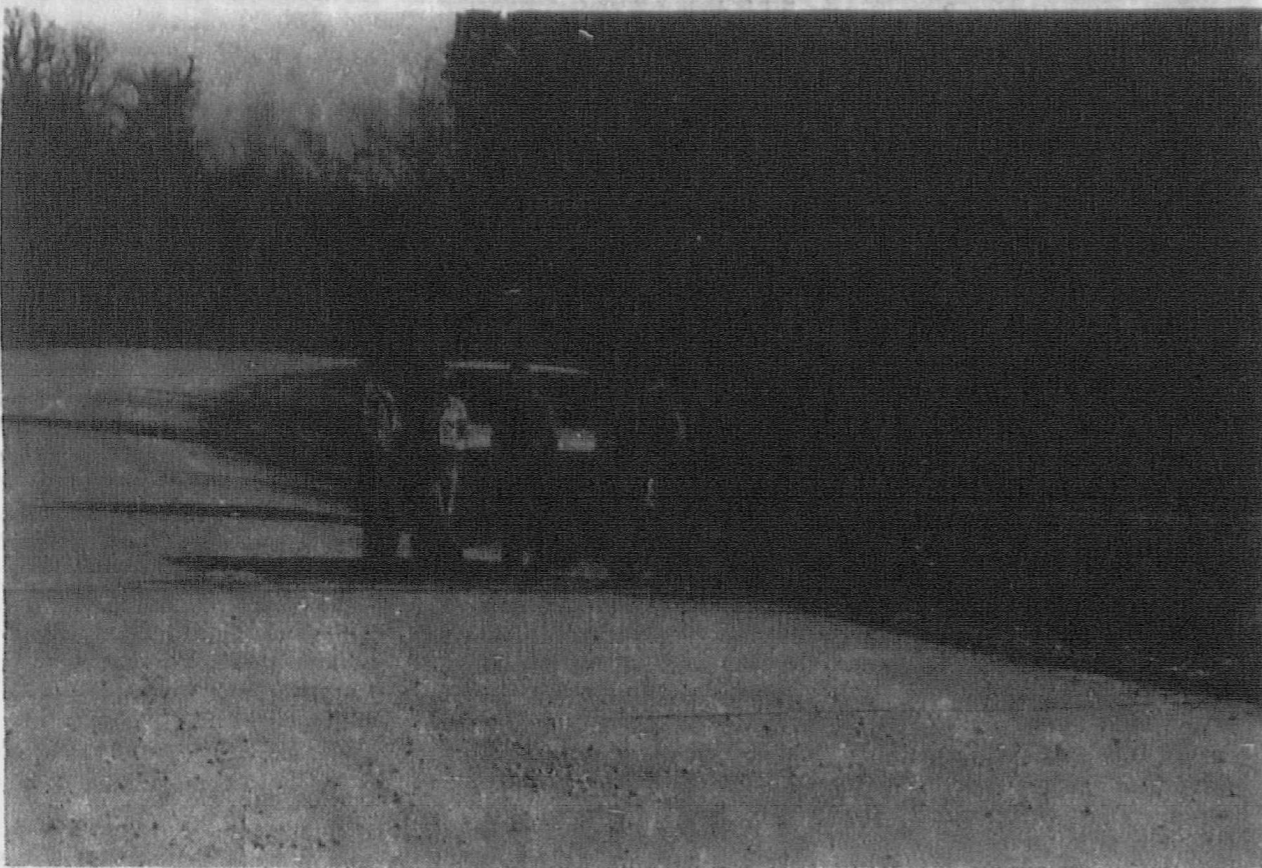
Pleasant Grove paving project
