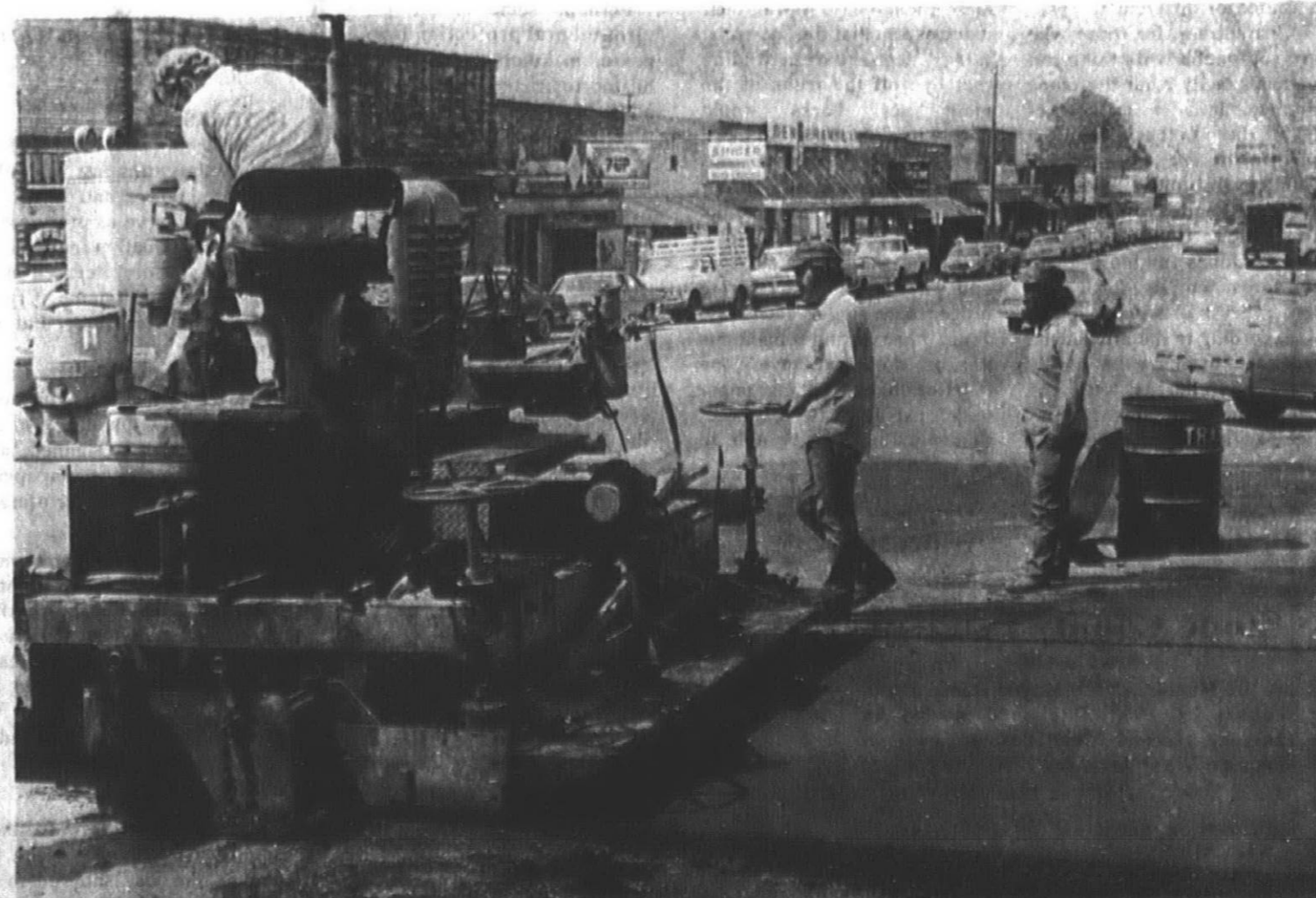
Courtsquare area paved
