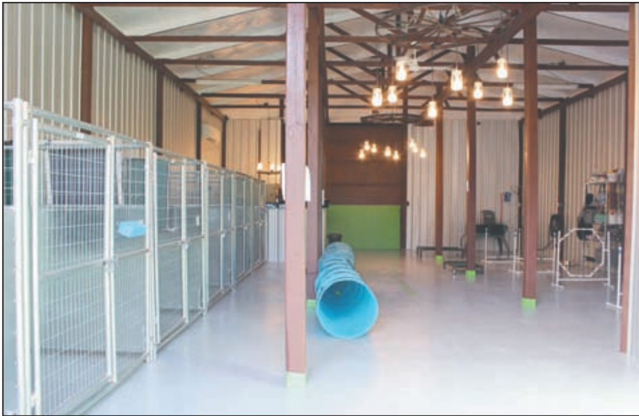
The interior of Country Pet Playground required extensive refurbishing of an existing metal structure. Kennels line one wall, with grooming and play area occupying the remainder of the space. Owner Karissa Shambarger said she may add a few small kennels for smaller dogs.
