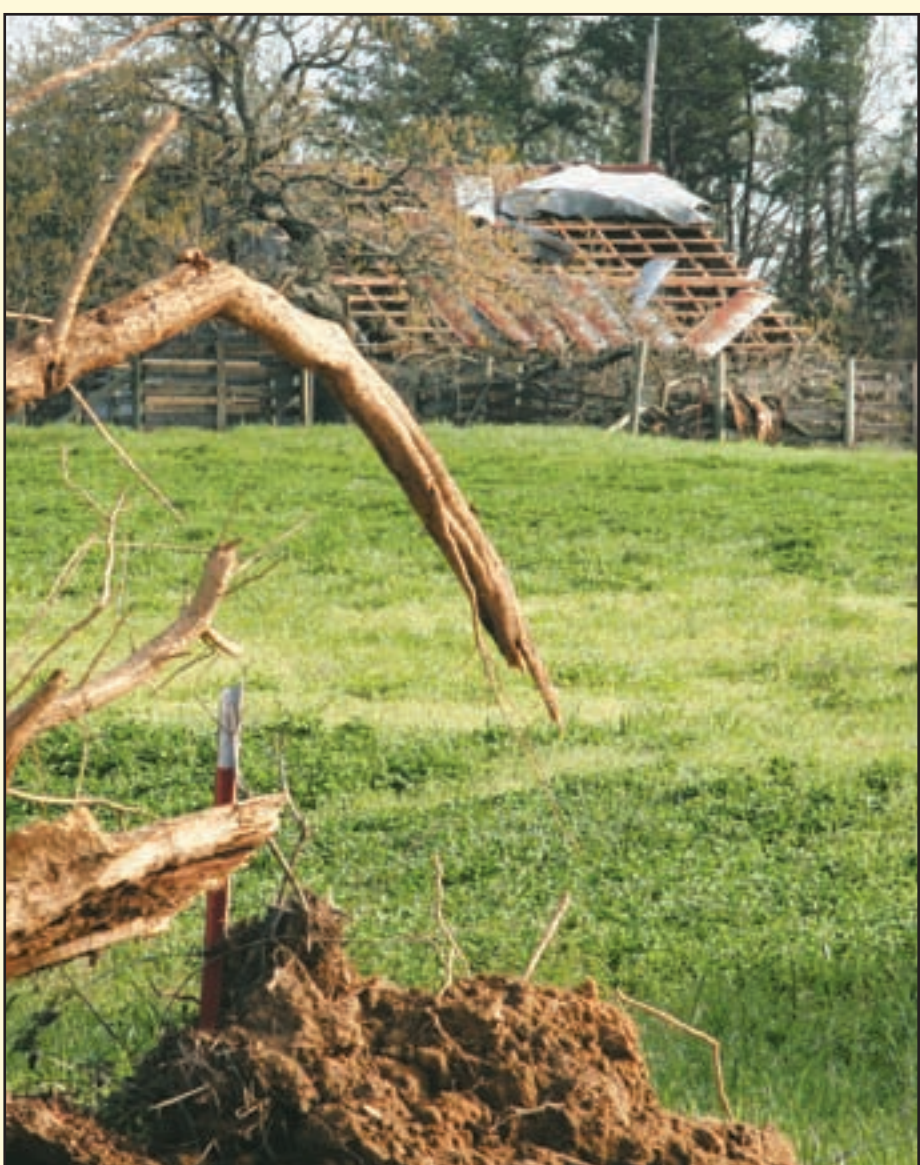
Trees were downed and structures were damaged on Happy Hollow Road.
