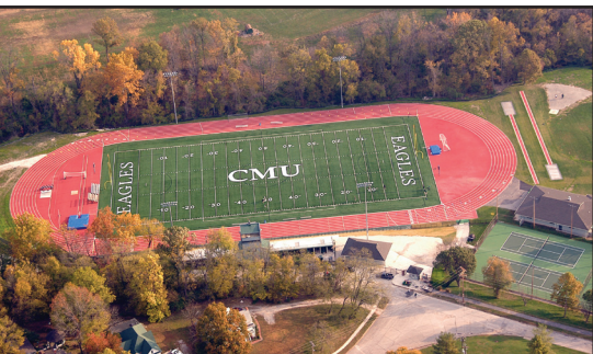
Aerial photo shows new Hairston 8-lane track and artificial turf on Davis Football Field, part of the athletic facilities upgrades made possible by the Campaign for Eagle Athletics.
