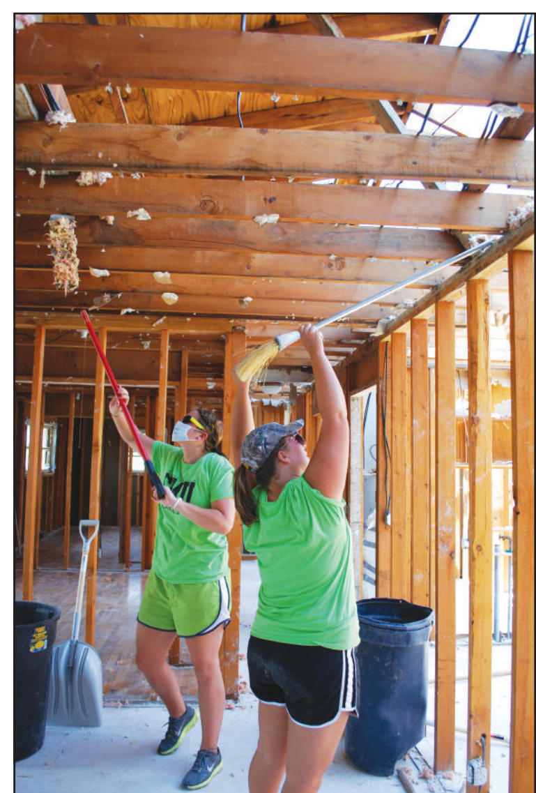
Two volunteers from Central Methodist University's mission group remove insulation from one of the homes damaged during the Joplin tornado. A group of more than 70 CMU students, alumni, faculty and staff helped with the relief effort during the one-day visit, working primarily around the grounds of Joplin High School.
