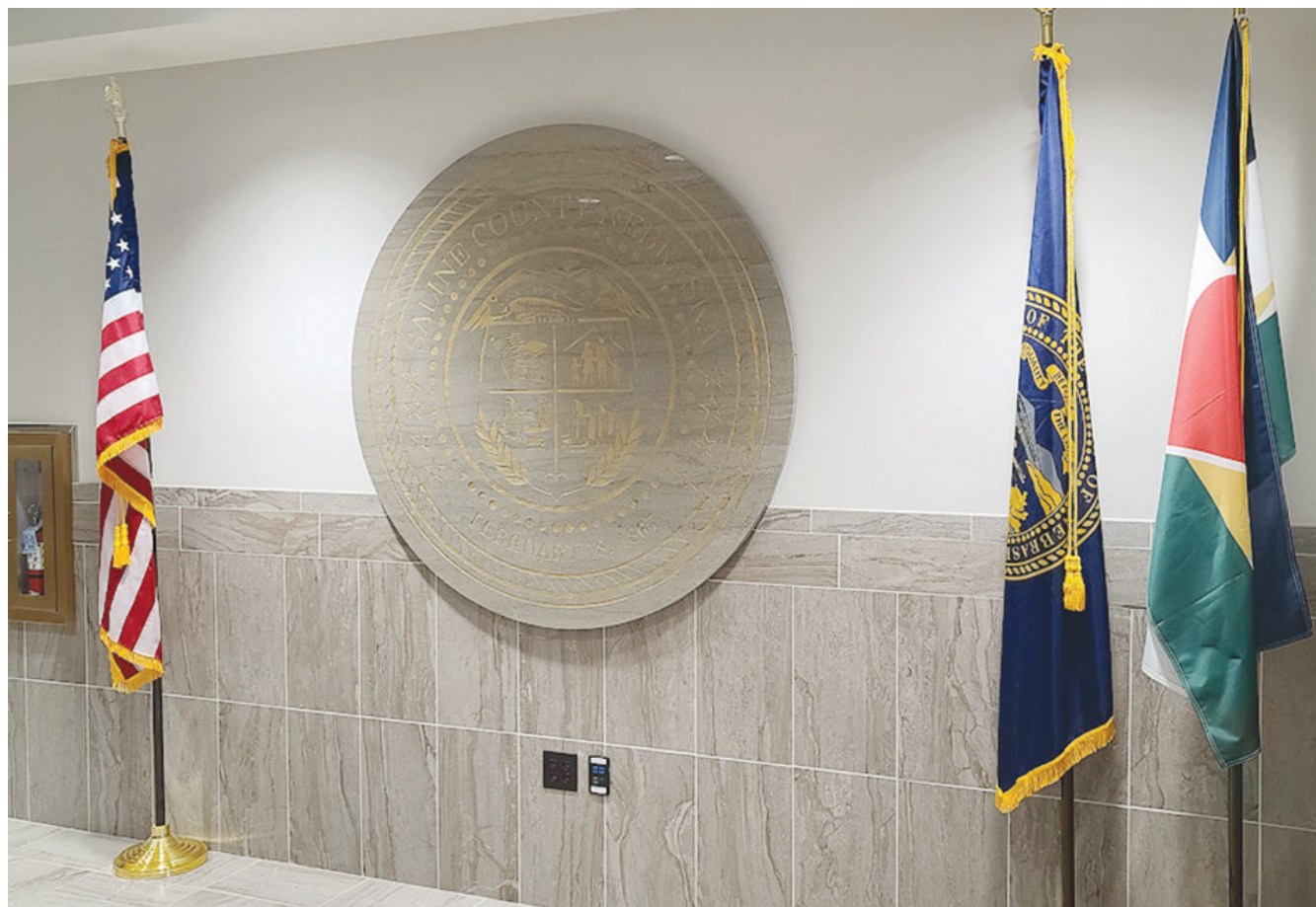
A concrete slab formed in the shape of Saline County's seal was attached near the front entrance of the courthouse in Wilber on Jan. 12. Pictured is the final result.
